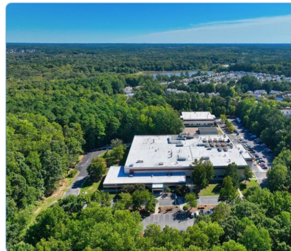
Raleigh, North Carolina facility
